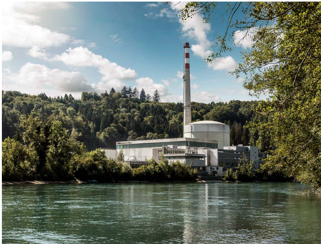
Figure 2: River view of Mühleberg NPP – Source BKW
