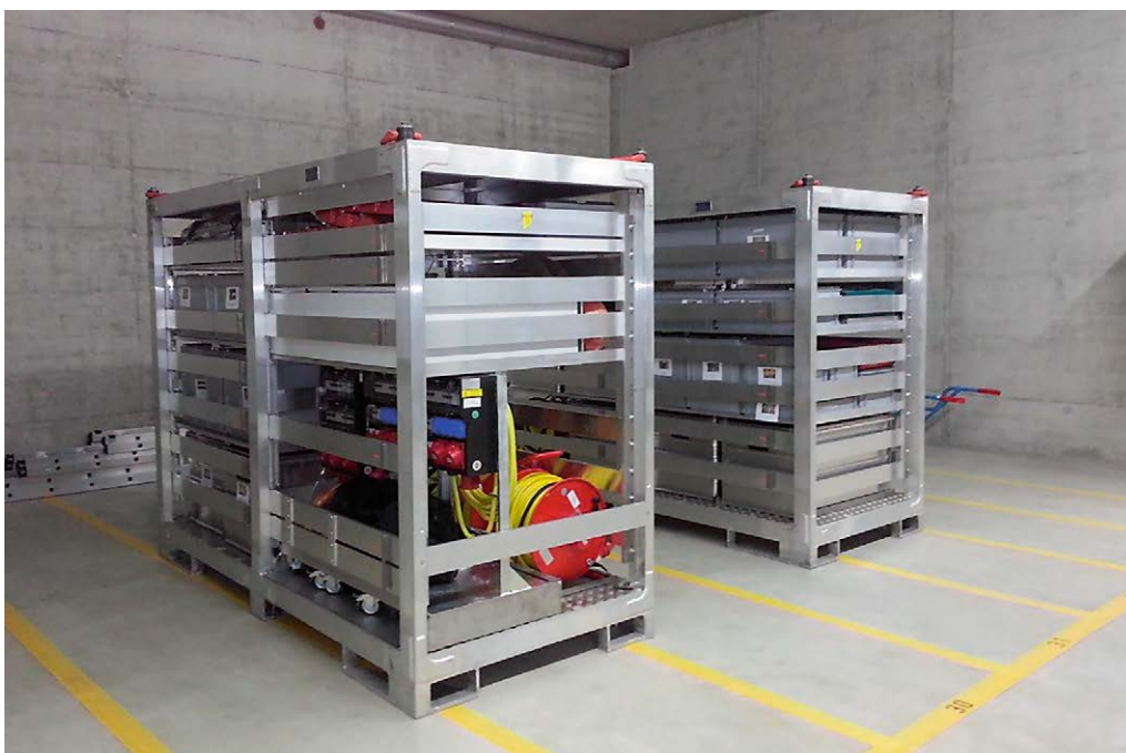
Figure 16: Storage Facility Reitnau – Source ENSI
