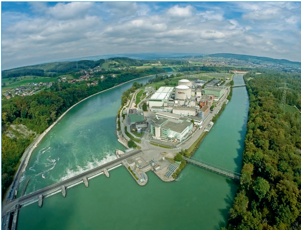
Aerial view of Beznau NPP – Source Axpo Power AG
