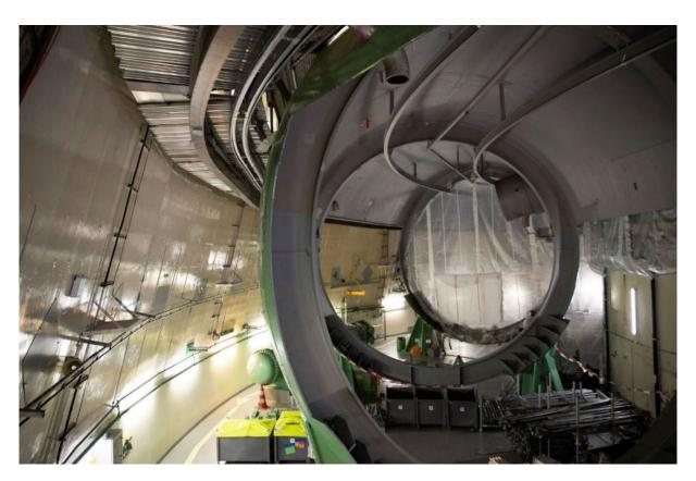
Figure 10: Reactor building – remaining support rings of the torus after completion of dismantling work Phase 1 (Source: BKW)
