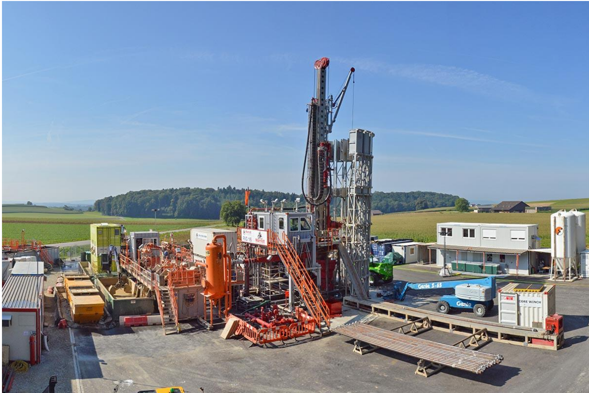
Figure 8: Nagra drilling site “Trüllikon-1” (Photo Nagra)
