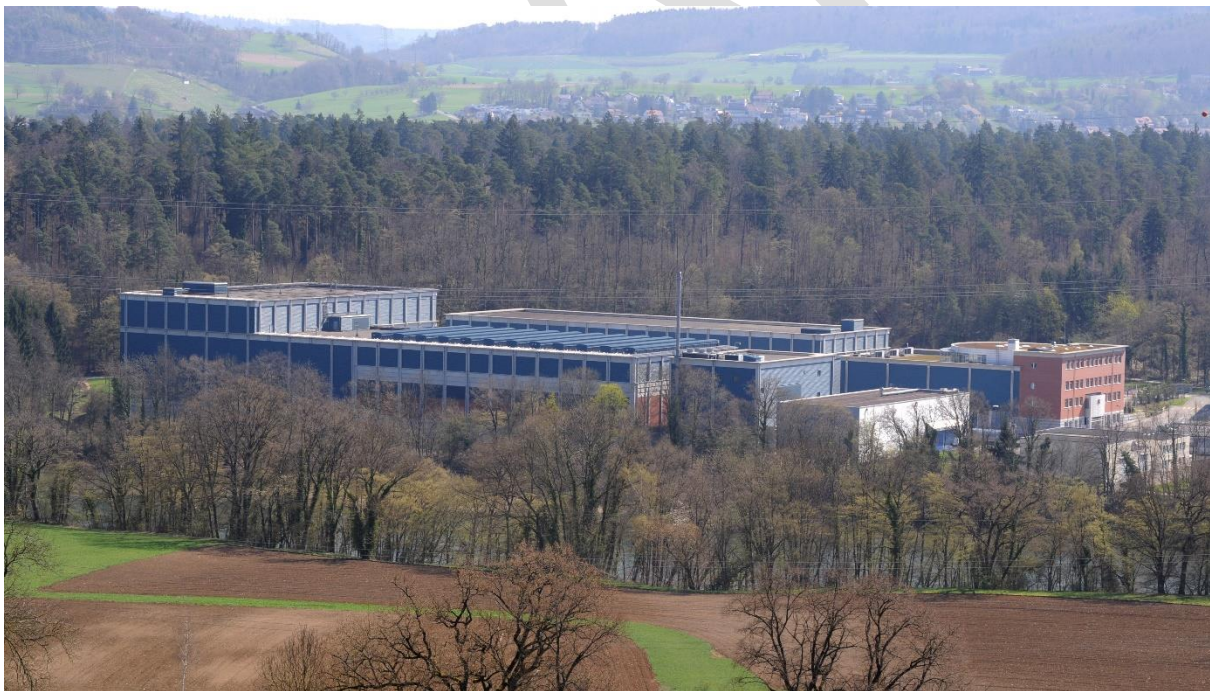
Figure 3: Central Interim Storage Facility of radioactive waste (ZZL) in Würenlingen. The facility is operated by the utility-owned company Zwiilag (Photo: ENSI).
