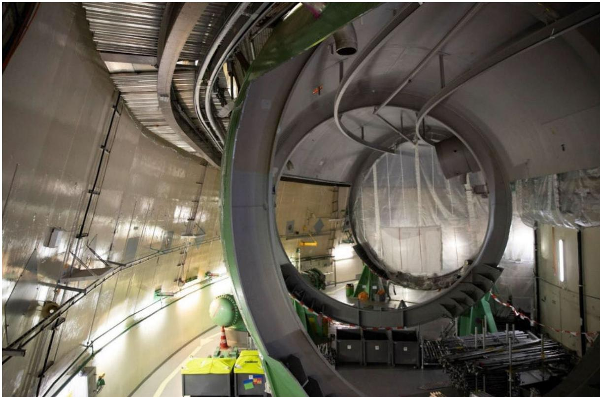
Figure 10: Reactor building – remaining support rings of the torus after completion of dismantling work Phase 1 (Source: BKW)
