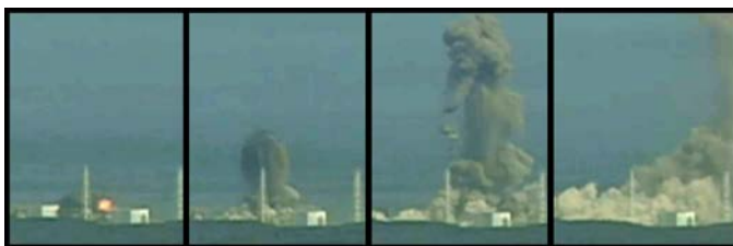
Figure 13 Explosion 20 Fukushima Daiichi Block 3; Standbilder: NTV Japan
